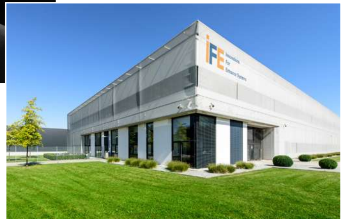
v The IFE facility in Kematen/Ybbs
